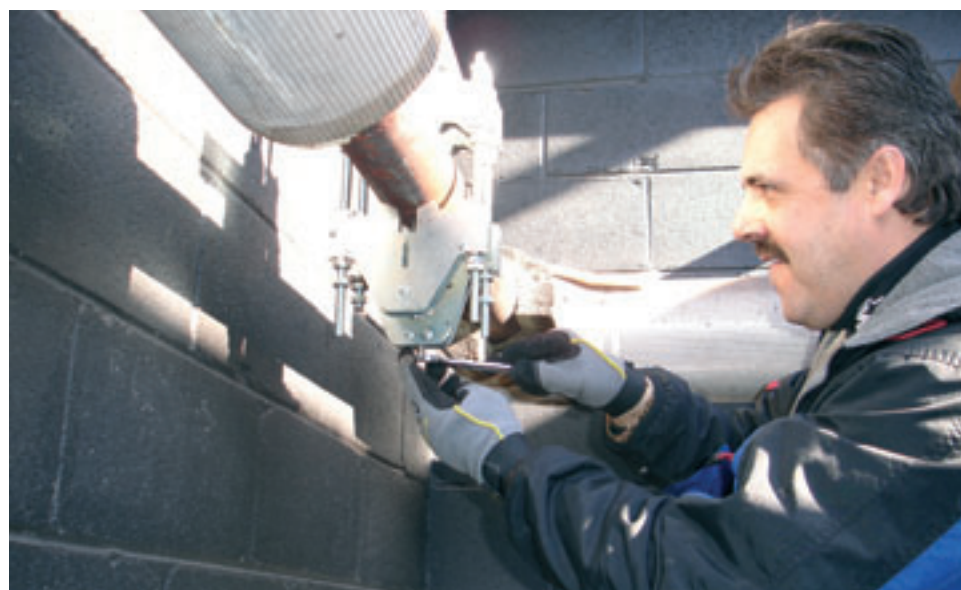
Installing the WavelInjector® at Tallant Industries
